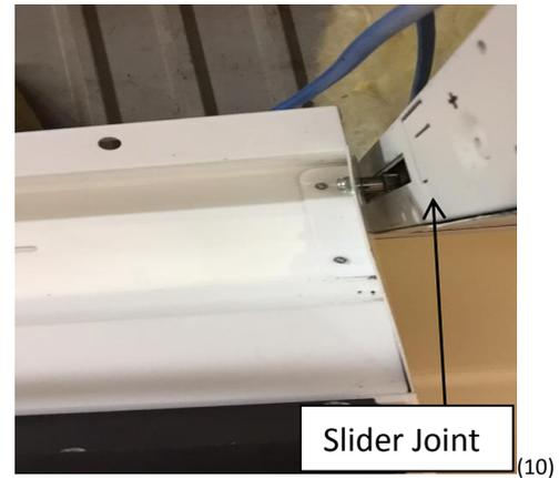
At this point, the fixture should be hanging at the end of the mounting bracket and should be parallel in the drop ceiling frame (not at an angle). With the fixture hanging from the ceiling, you are now ready to install the power connector. (Image 11)
