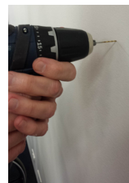
1.5mm (1/16") drill bit for mounting on wood, wood studs or metal
